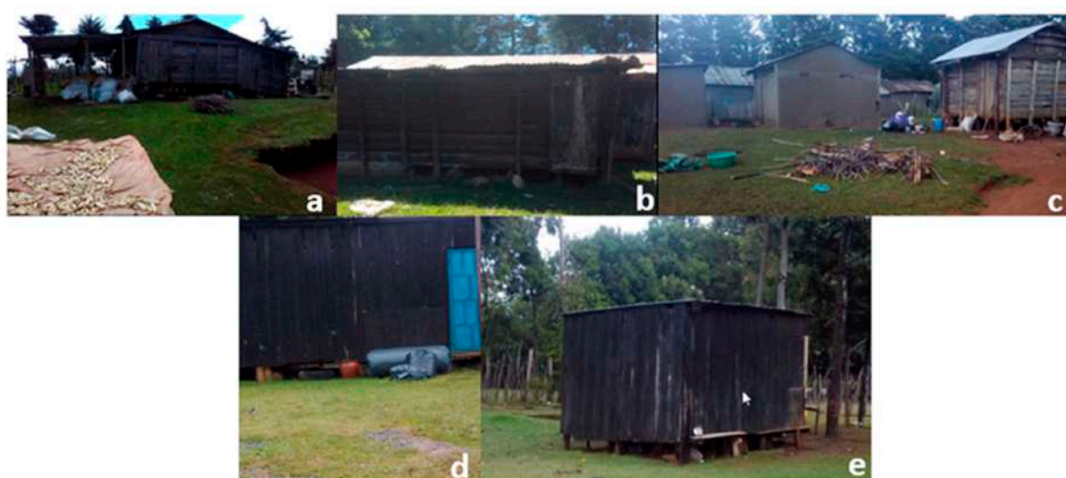
Figure 5. Illustration of the different storage structures within the Rift Valley. (a–c) semi-permanent wooden granaries built with minimal elevation from the ground; (d,e) semi-modern wooden granaries raised slightly from the ground to deter entry of rodents and crawling pests.
