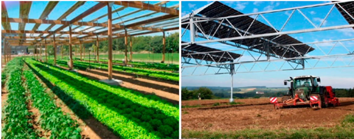
Figure 4. (a) Panels installed at the height of 4 m in Montpellier © Dupraz, (b) Panels installed at the height of 5 m in Germany © Fraunhofer ISE [33].
