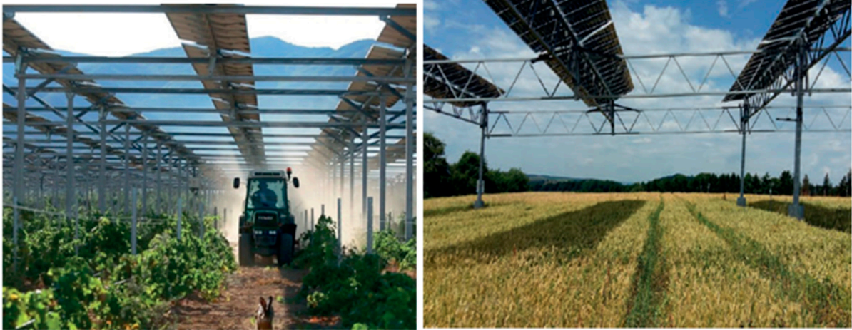
Figure 6. Spacing between rows of panels allowing movement of farm machinery under the PV panels © Fraunhofer ISE [44].
