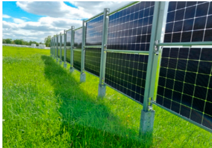
Figure 8. Vertical agrivoltaic installation with bifacial modules in Sued [62].
